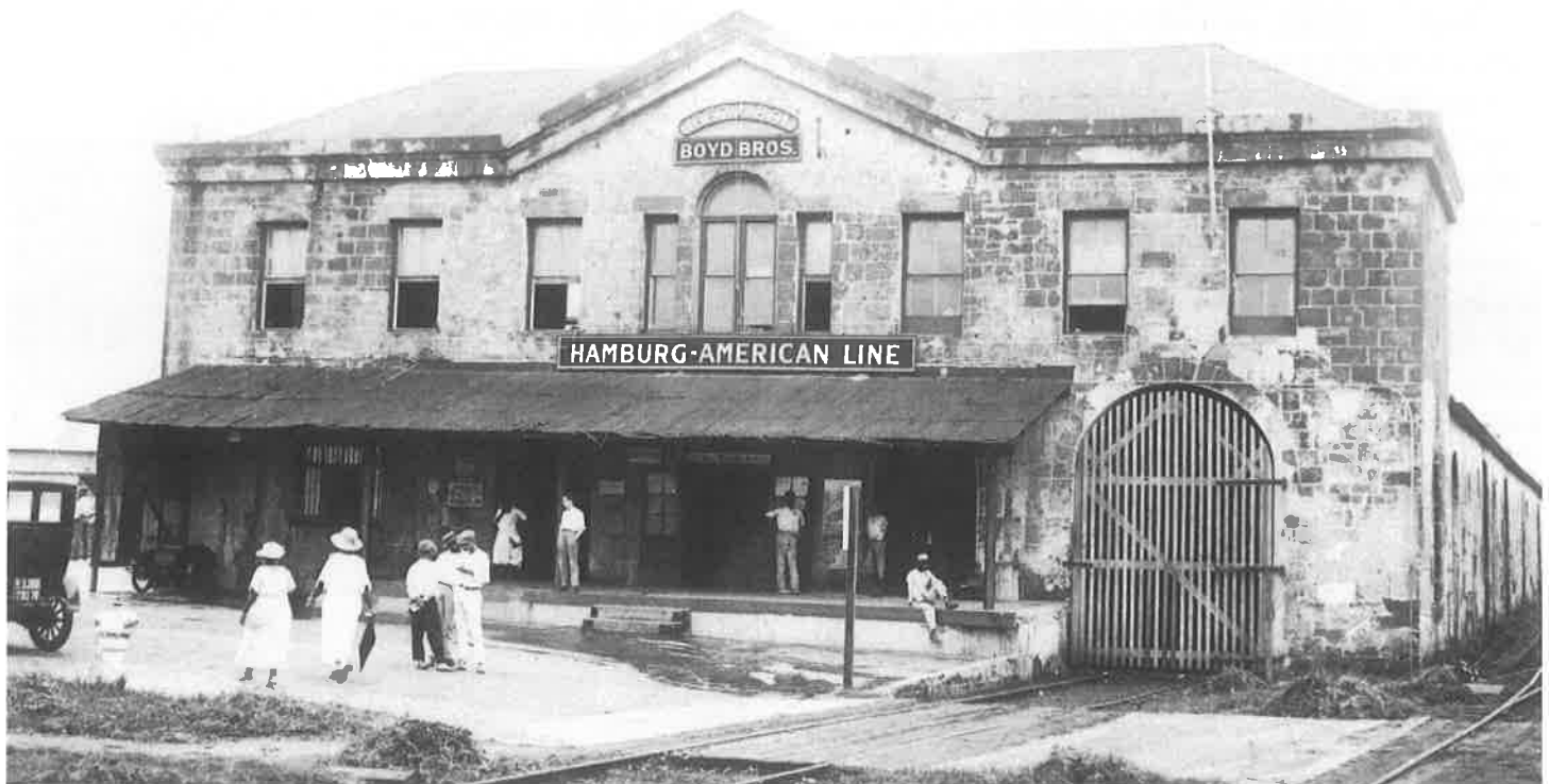
Boyd warehouse in Colon
